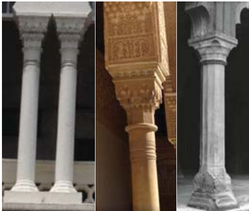
Fig. 11 (a) Muqarnas capital seen on Kuala Lumpur Station (b) also similar to columns at Alhambra Palace, Spain and (c) Taj Mahal, India
