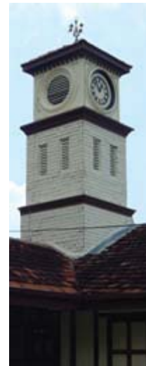
Fig. 15 Alor Setar Station's clock tower
