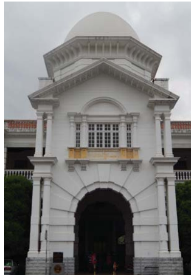
Fig. 20 Voussoir round arches in Ipoh Station
