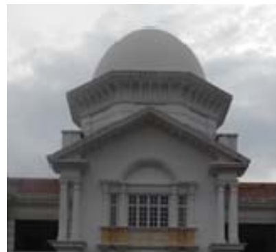
Fig. 4 Main dome located at the centre of the building
