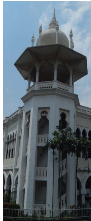
Fig. 12 Staircases tower at Kuala Lumpur Station
