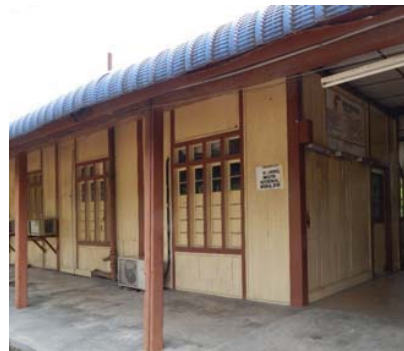
Fig. 21 The upper window part has been changed into glass to suit the usage of the air-conditioned
