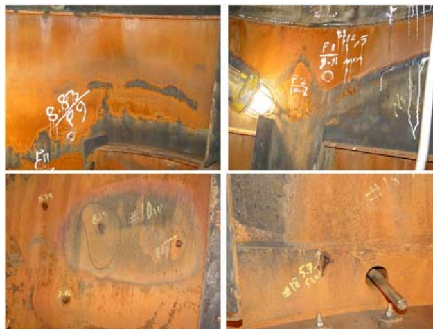
Fig. 3 CORROSION on Different Side of Shell(Top left to right ,Tray 9, tray 8, Bottom left to right ,Tray 10, Tray 18)
