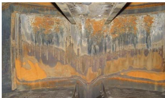
Fig. 1 Corrosion on shell on vapor area
