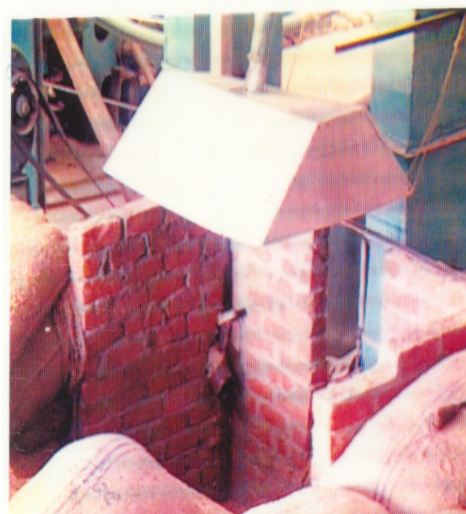
HOOD OVER PADDY SILO
