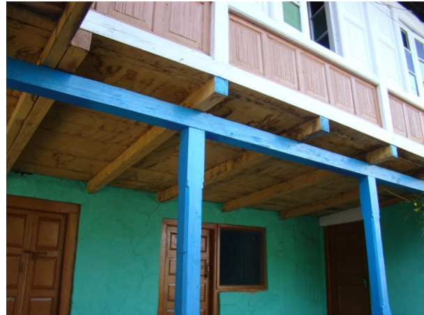
Fig. 6 Timber flooring and cantilevered balcony
