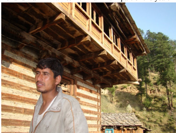
Fig. 5 Traditional 'Kath-khuni' wall construction with timber & stone
