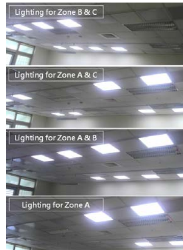
Fig. 11 Controls for dedicated lighting zone
