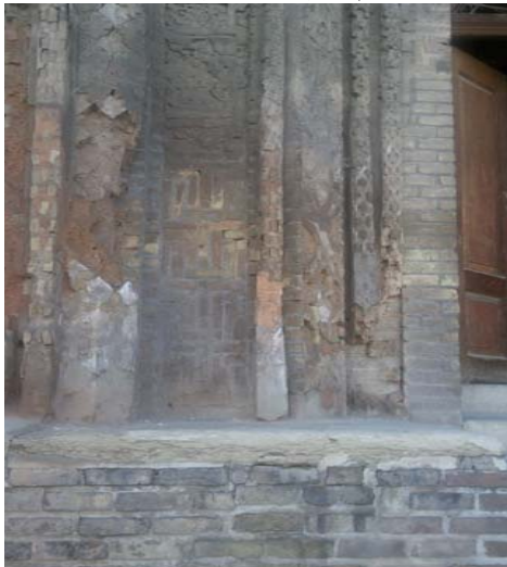
Fig. 5 penetration of moisture into the pores of the building and freezing between the bricks which shatters them in cold regions (Alavian dome, Hamadan, Iran)
