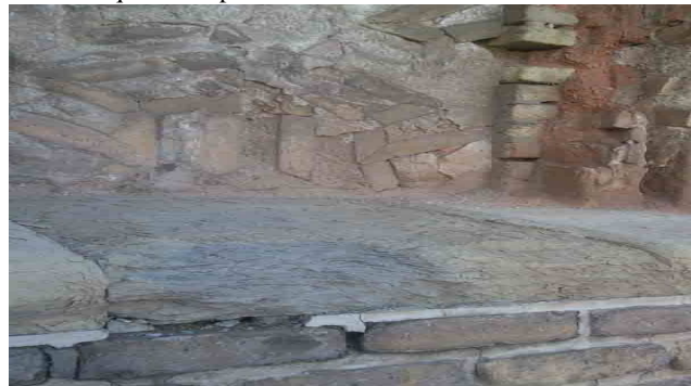
Fig. 3 Decomposition of stones due to acid rains
