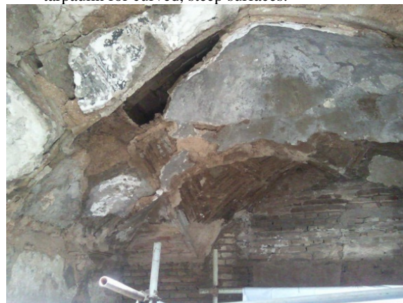
Fig. 7 Damages due to descending moisture (Vakil Bath, Shiraz, Iran)
