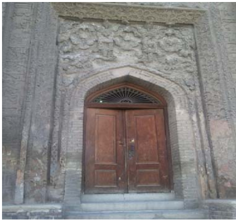
Fig. 4 Moisture along with fluctuations in temperature can lead to disintegration of the façade (plasterwork) in cold regions (Alavian dome, Hamadan, Iran)
