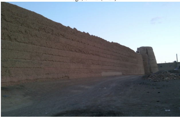
Fig. 2 destruction and erosion of an earthen building due to climatic factors (Damab castle, Isfahan, Iran)
