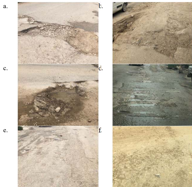
Fig. 1 Distress identified from Tripoli's roads (a. transverse crack, b. raveling (loss of coarse aggregates), c. potholes, d. bleeding and rutting, e. raveling and bleeding, f. fatigue/alligator cracks)
