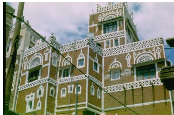
Fig. 9 Traditional house in Sana'a city (mud bricks construction)
