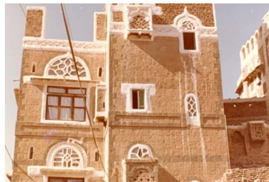
Fig. 10 Traditional house in Sana'a city (stone construction)
