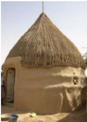
Fig. 6 Mud and reed hut, Tihama, Yemen [7]
