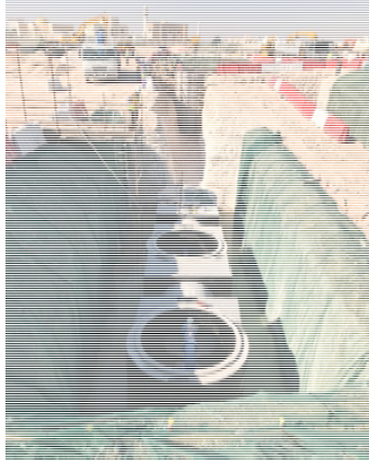
Fig. 18 Construction of three manholes for wellhead assembly
