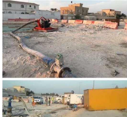
Fig. 22 Water pumped into the injection well from EFA pond at Site 10, FPS14
