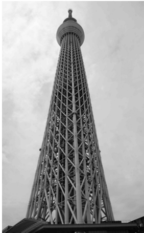
Fig. 10 Tokyo Skytree Tower
