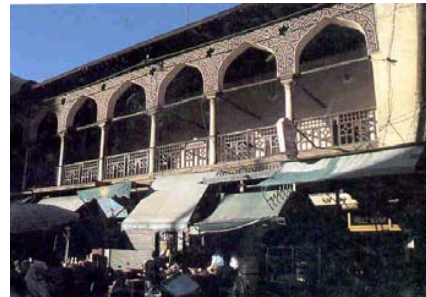
Fig. 7 The Agency and Mosque of Al-Shorbaji
