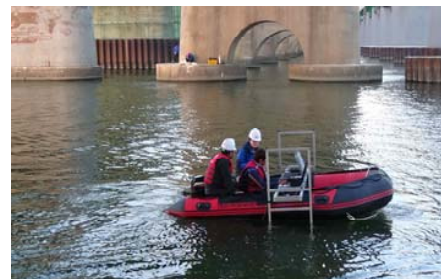
Fig. 2 Underwater structure survey using SSS
