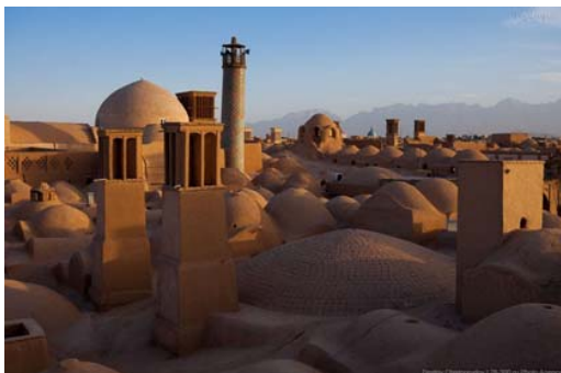
Fig. 1 A view of a traditional pattern in Yazd (city in center of plateau of Iran). Domical roofs minimized possibility of heat exchange in dry and hot regions [10]
