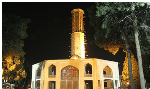
Fig. 2 Windward is one of the key elements of Iranian architecture. This is the Dolat Abad wind ward and the highest one in the world [11]
