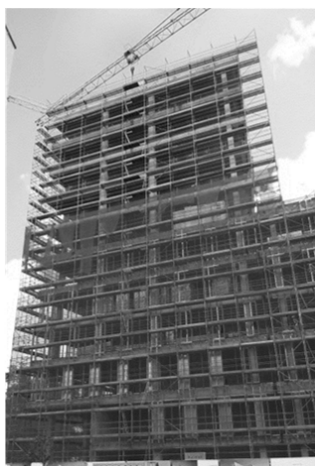
Fig. 1 A view of the scaffolding
