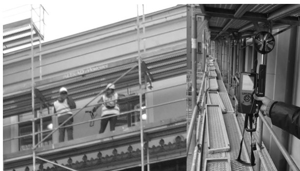
Fig. 3 The measurements on the scaffolding
