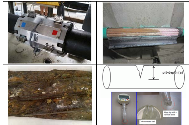
Fig. 1 Inspection procedure for corroded tendon
