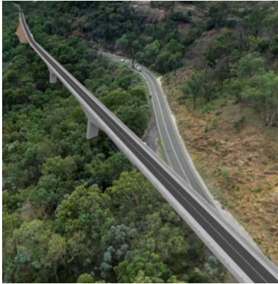
Fig. 7 Completed bridge in relation to existing road
