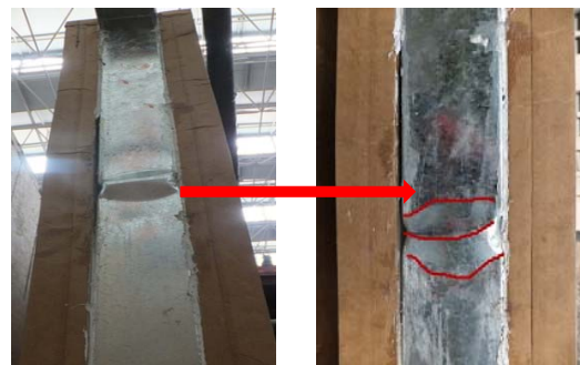
(b) Local buckling of W-2 CFS
