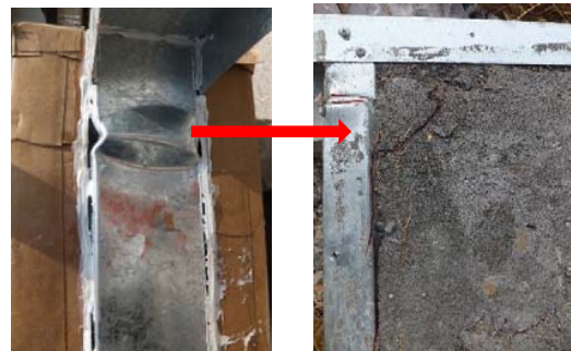
(c) Local buckling of W-3 CFS
