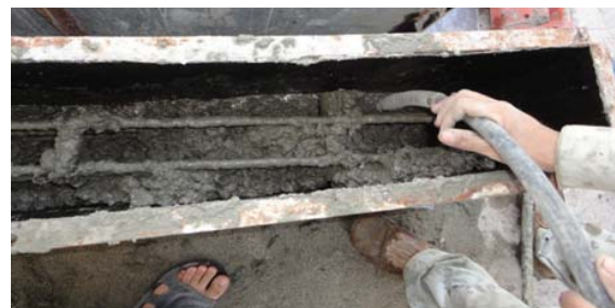
Fig. 4 Compaction of concrete in moulds with vibrator
