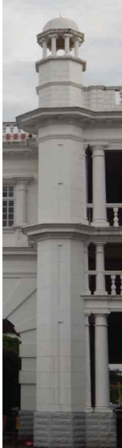
Fig. 13 Minaret tower at Ipoh Station
