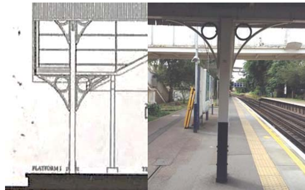
Fig. 8 (a) shows similarity on columns with spandrels at Taiping Station, Malaysia with (b) Kew Garden Station, Britain
