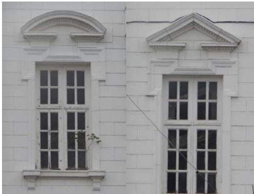
Fig. 23 (a) Circular and (b) triangular pediment as a window trims in Ipoh Railway Station
