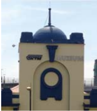
Fig. 6 Dome located on top of the tower mounted with finial
