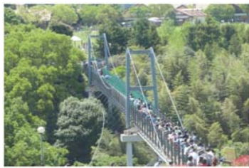
Fig. 12 Existing suspension pedestrian bridge
