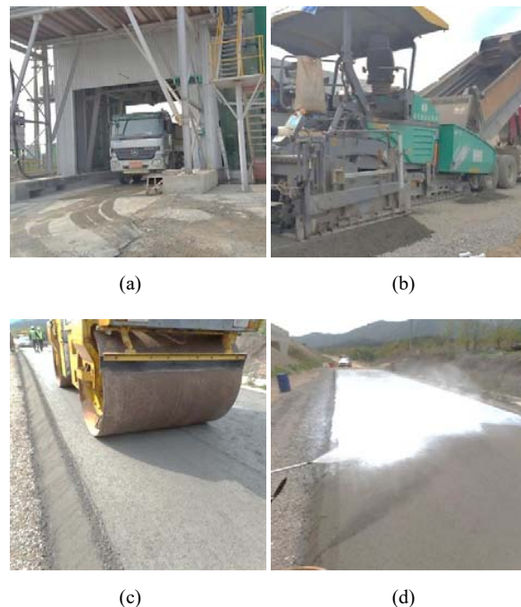
Fig. 2 Construction process of RCCP (a) Mixing and transportation, (b) Paving, (c) Compaction, (d) Curing
