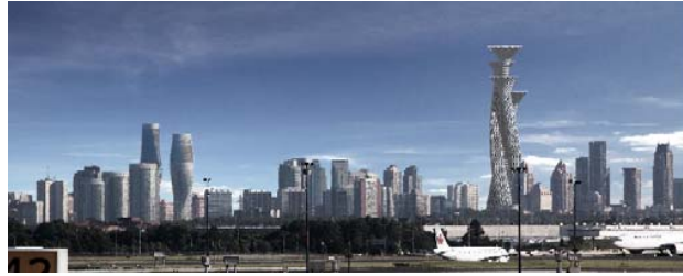
Fig. 4 3Ts in the Mississauga skyline
