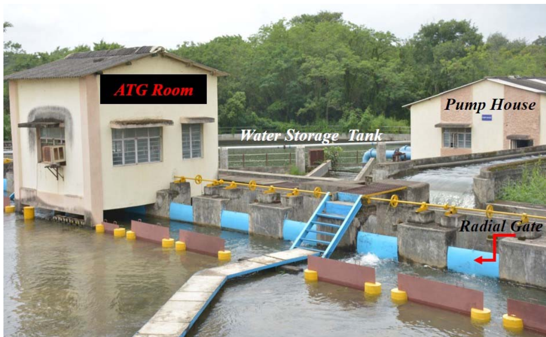
Fig. 4 Automatic tide generation system
