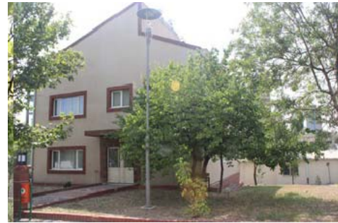
Fig. 7 (b) The appearance of the western façade of the sample building
