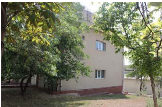
Fig. 7 (a) The appearance of the eastern façade of the sample building
