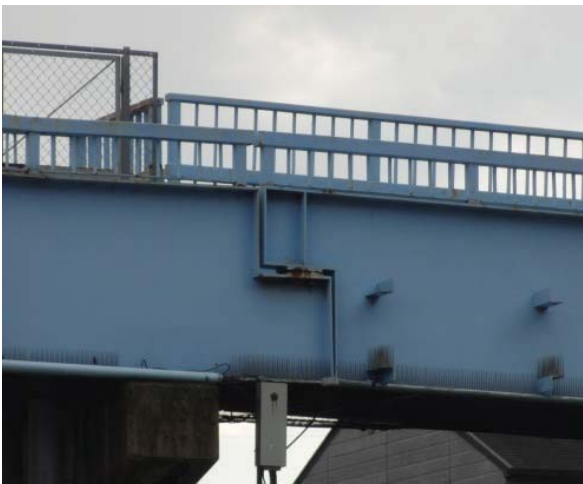
Fig. 2 Hinge connection at middle bridge pier
