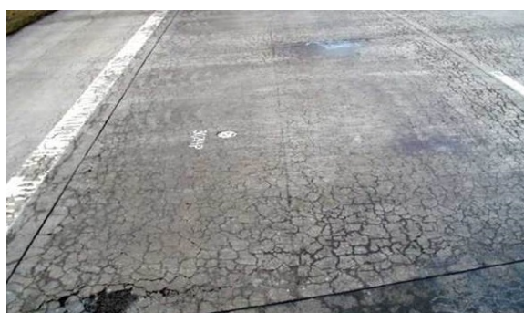
Fig. 1 Damage of top layer of the concrete road with RCA due to ASR
