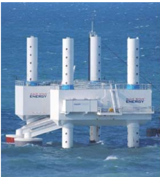
Fig. 10 Wavestar prototype at Hanstholm [18]
