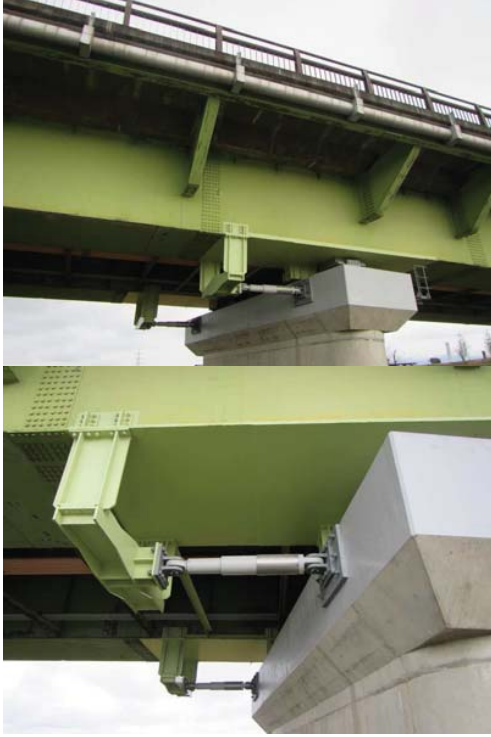
Fig. 2 Earthquake-Resistant Dumpers for Bridge
