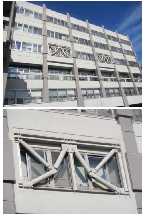
Fig. 1 Earthquake-Resistant Dumpers for Building
