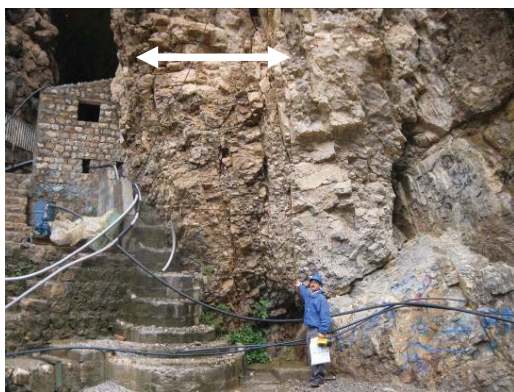
Fig. 5 Fractured zone of CBF
