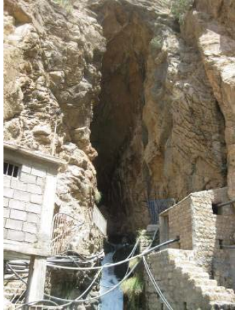
(a) Before plugging
