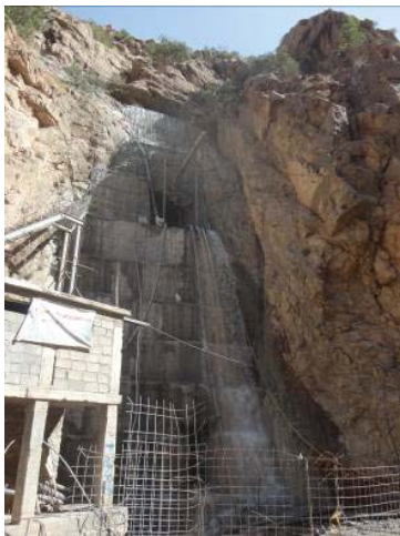
(b) After plugging
