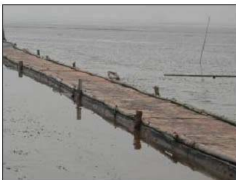
Fig. 3 Complete floating bridge
