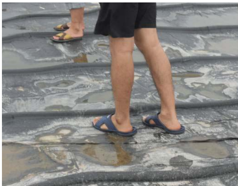
Fig. 10 Ground in half way of foundation treatment
