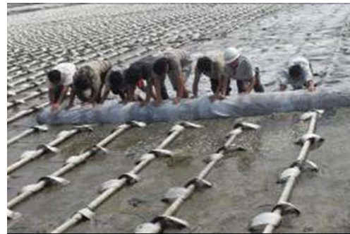
Fig. 7 Working photo of laying vacuum membrane
