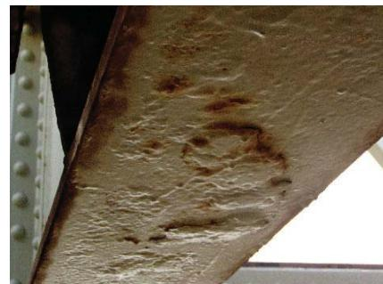
Fig. 1 Appearance of Under-film Corrosion
