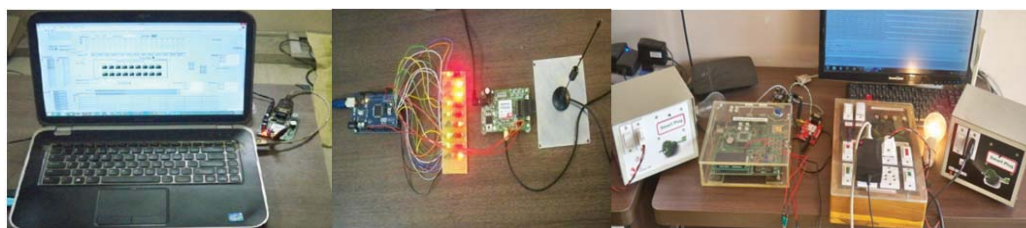
(c) Complete setup (Server, programmable load and HAN1)
