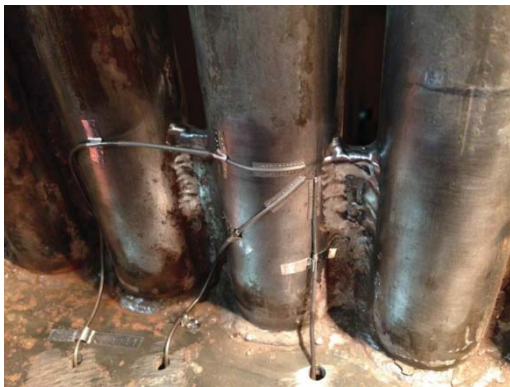
Fig. 3 Strain gage installation on boiler tubes
