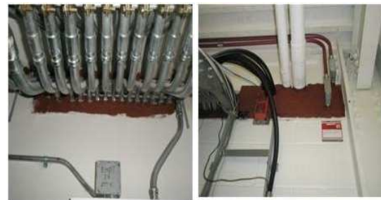
Fig. 9 Fire penetration protection system
