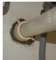
Cracks seal to avoid standing water and pests
