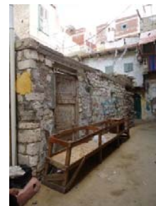
Fig. 4 Ruins of Sayied Darwish historic building
