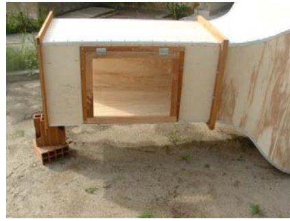
Fig. 5 Construction of the section of rehearsals
