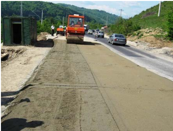
Fig. 1 Roller compacting
