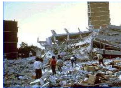
Fig. 4 Mexico City Earthquake: Collapse of an 8 level building in 1985
