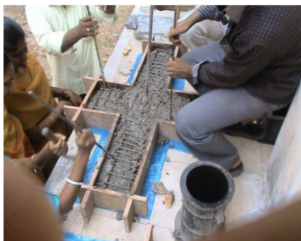
Fig. 9 Casting of beam column joint
