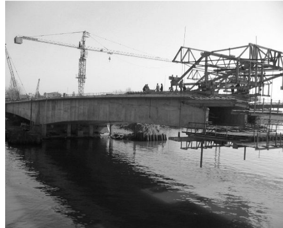
Fig. 1 Box bridge constructed by free-cantilever method in study
