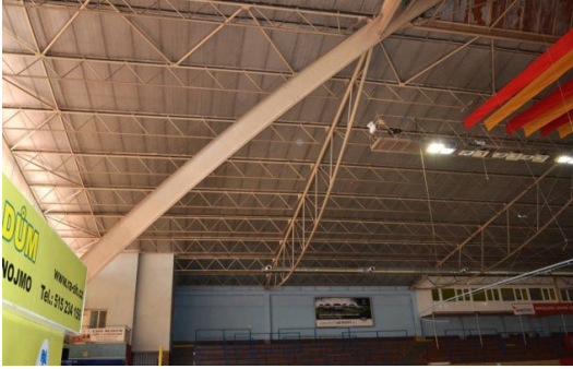
Fig. 7 Part of tested structure: truss main roof girders, truss purlins, bracings, arch main girders
