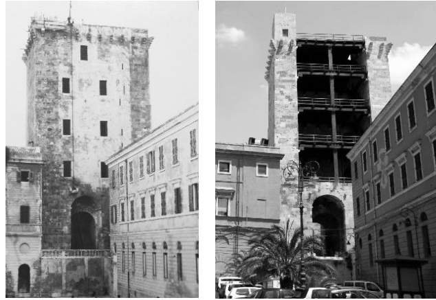
Fig. 14 San Pancrazio Tower before and after the wall demolition
