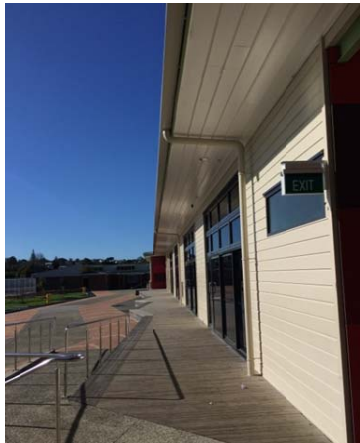
Fig. 3 One-story building with light rain screen wall
