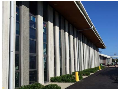
Fig. 1 Maths Building with precast insulated concrete panel walls
