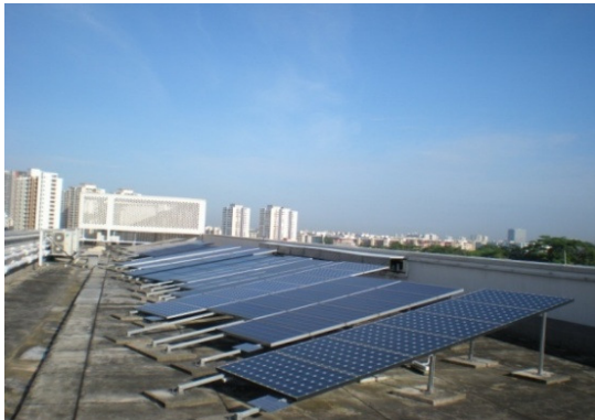
(b) After installation of PV systems
