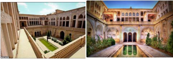
Fig. 7 The Sunken garden in Abbasian house, Kashan, Safavid era
