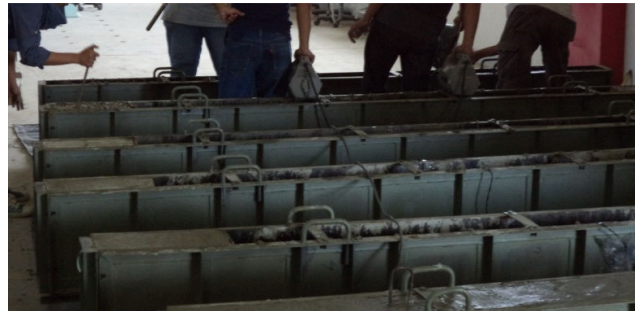
Fig. 3 Casting of Specimens
