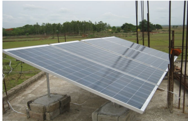
Fig. 8 Rooftop PV system
