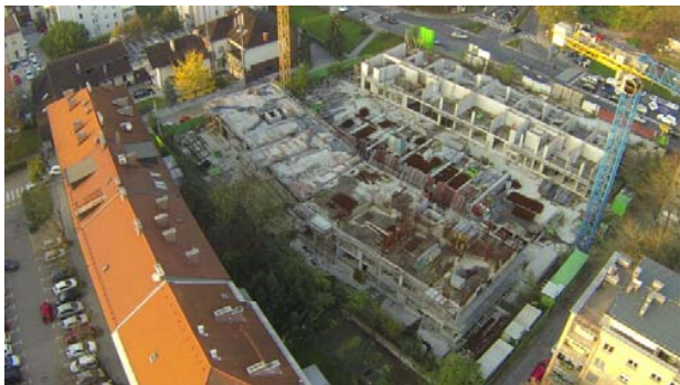
Fig. 8 Abandoned construction site in Ljubljana [15]
