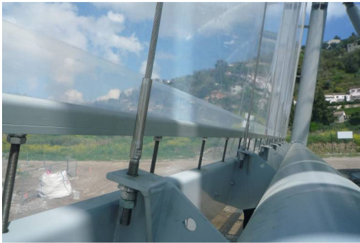
Fig. 13 Picture of prototype – Fixation detail seen from inside
