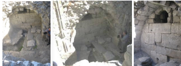
Fig. 7 Fountain's north façade
